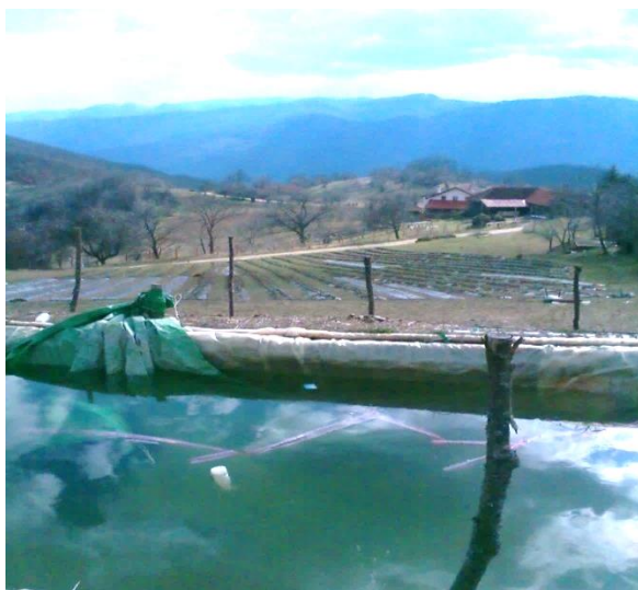
Improvised water tanks
